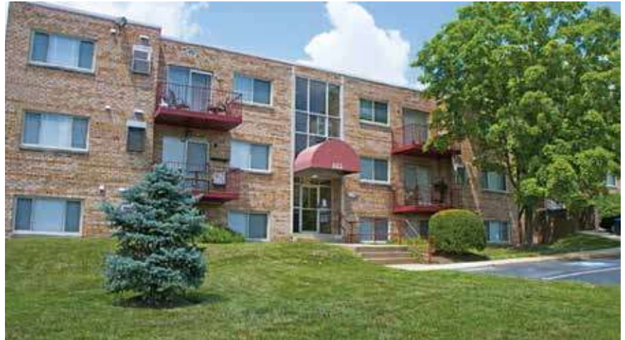
M.TEB helps DC's Hilltop Apartments remain affordable permanently.
